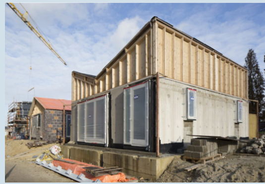
Figure 3a - Examples of harvested materials from the 10-story housing block (on building, product and material level) to be used in new construction (Dusseldorf 2019).
